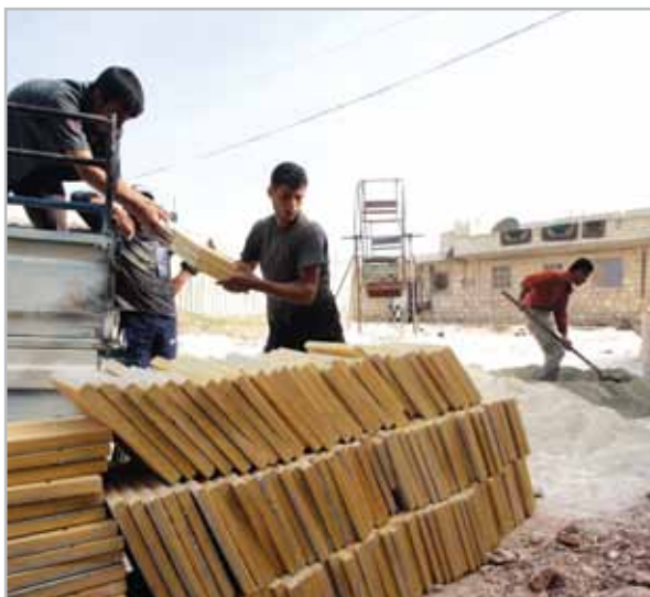
Reconstruction site at the Neirab Camp , Syria
